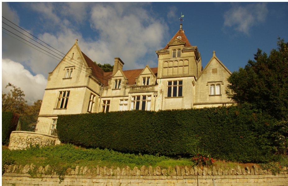
Figure 4: Rodborough Court in course of restoration 2021. Photo Ian Johnson.
