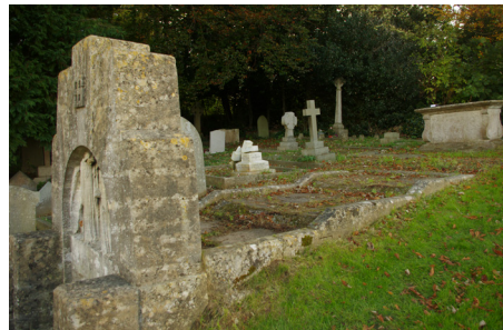
Figure 3: The mausoleum today showing the extent of the vault Photo Ian Johnson
