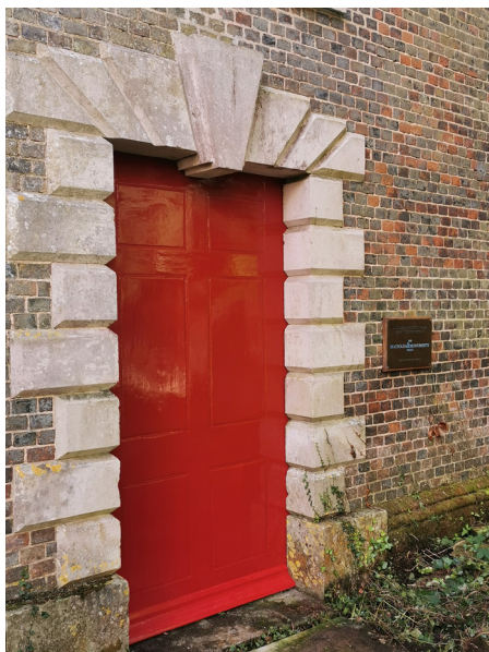
Figure 6: repainting the door at the Heathcote mausoleum in Hampshire
