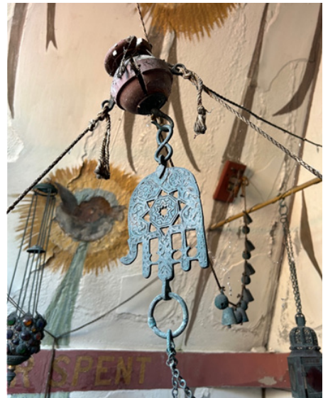
Figure 5: Hamsa hand suspended from wooden central boss which has become detached from the ceiling.
