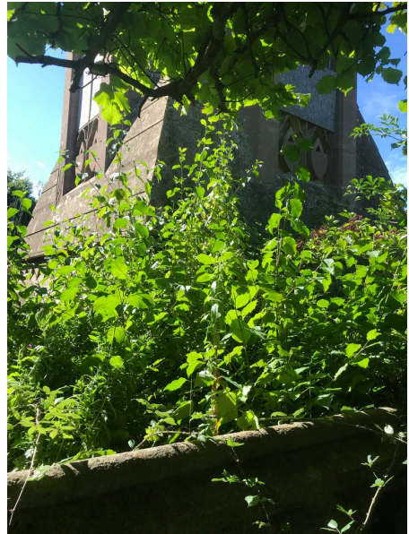
Figure 3: The mausoleum is overgrown.
