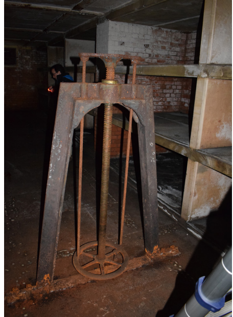
Figure 9: Newcastle vault showing one of the screw jacks for raising the vault slab, photo courtesy of Skillington Workshop Ltd. with permission of the Churches Conservation Trust
