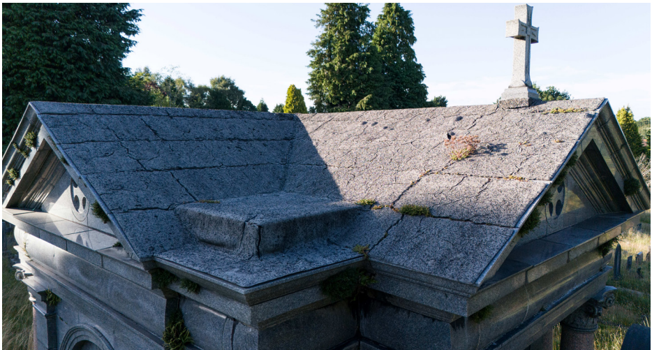
Figure 2: Roof of the Hogg Mausoleum
